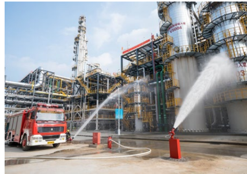
Yangnong Ruiheng conducted an drill to validate emergency plans before trial production of new plant
